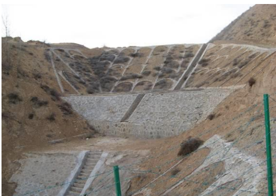
K46+550 弃土场坡面防护
