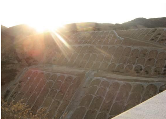
K52+800 弃土场坡面防护
