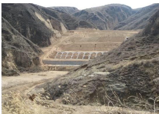
K62+000 弃土场坡面防护
