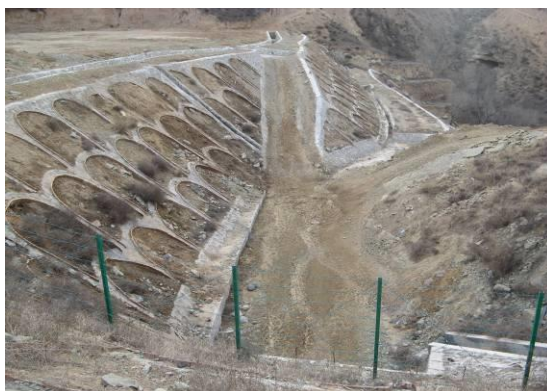
K48+900 弃土场坡面防护
