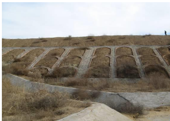
K42+000 弃土场拱形骨架护坡
