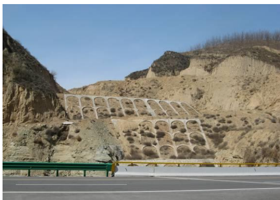
K58+200 弃土场坡面防护
