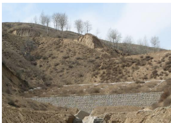
K56+600 弃土场砌石挡墙
